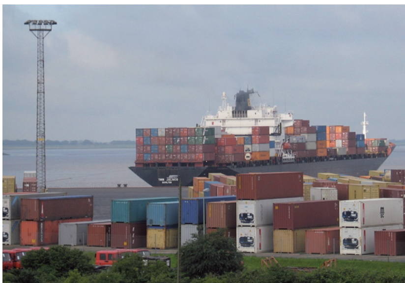
The linking of water – road – rail will become increasingly important
